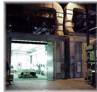
Paint booth at Letterkenny Army Depot, Pennsylvania
